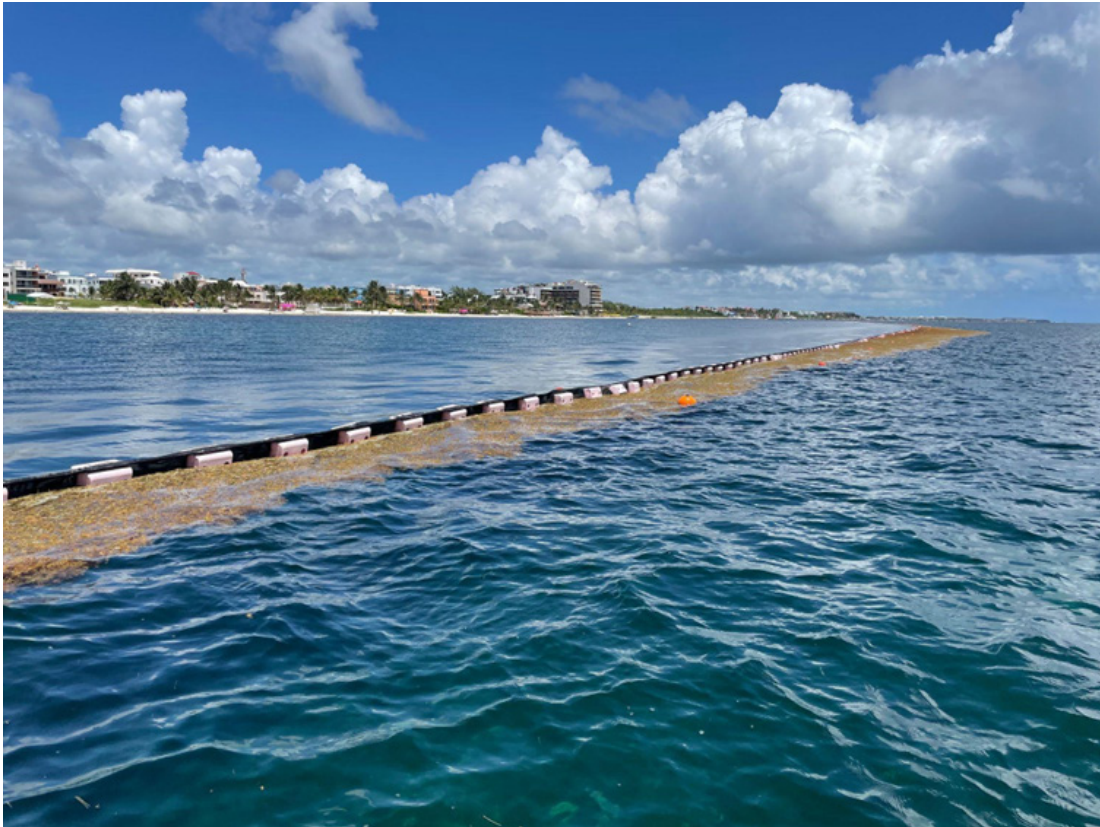
Barriers, as seen here in the photo, are installed in front of hotel beaches to keep the algae away. It does not, however, hinder the algae from accumulating behind the barrier. These barriers must be cleaned and maintained regularly to be effective, which is costly. Photo credit: Laura Otto.
